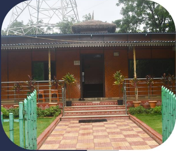
TSFDC Office Bamboo House
