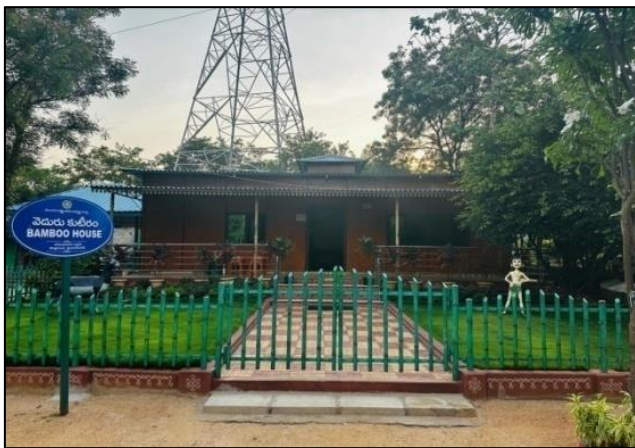
TSFDC Office: Bamboo House
