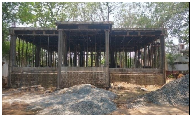
Construction of Divisional office Building
